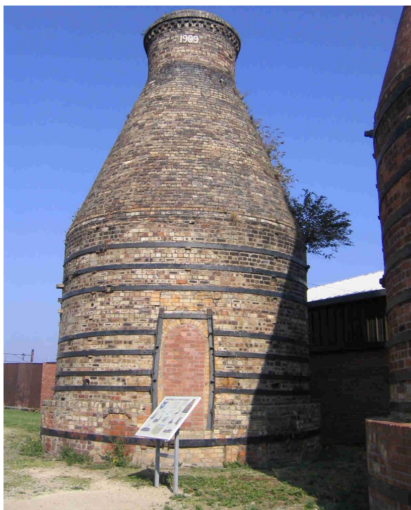
The kiln photographed in 2005 with plants growing out of its structure. Work on rebuilding is due to begin in the new year.
